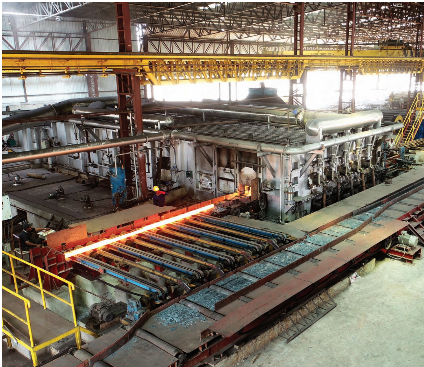
VIJAY SHRI STEEL Plant at Shivaraj, Kapilvastu, Nepal
